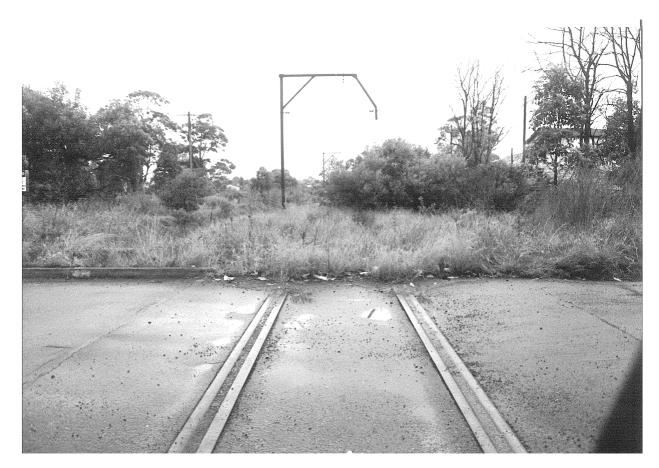
Figure 4 - Tracks filled with waste and disappearing into undergrowth at Enfield site with abandoned overhead electrification standard.<sup>225</sup>
